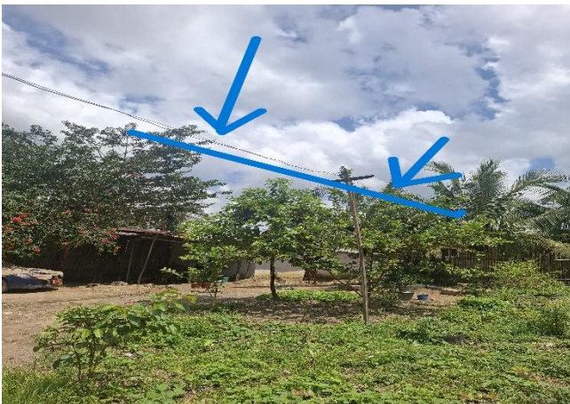
A service line passing through a is causing fluctuations during coconut tree thunderstorms or strong winds.
